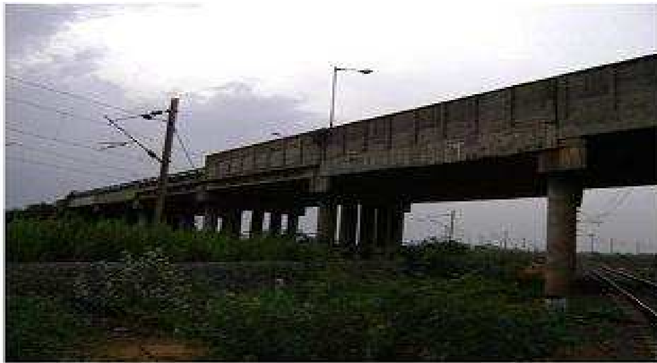
4.2 Kms from Port Gate Attipattu Rail Over Bridge
