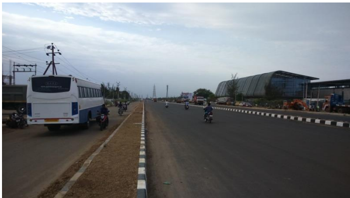
North side of Oragadam ⇒ Almost widening done
