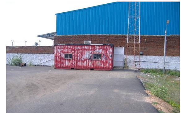
Pass Section in the Parking Yard
