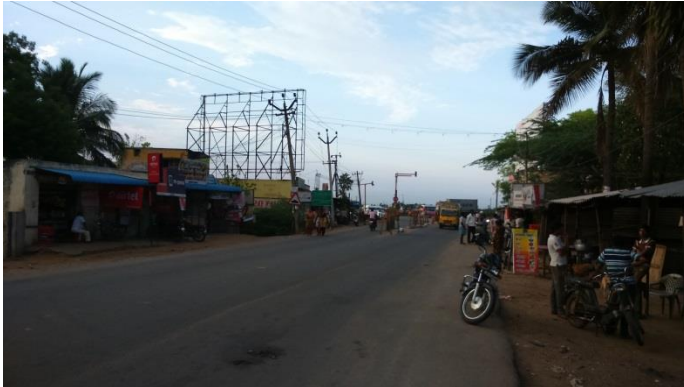
Crossing with SH57 - NH4 ⇒ Not started widening yet
