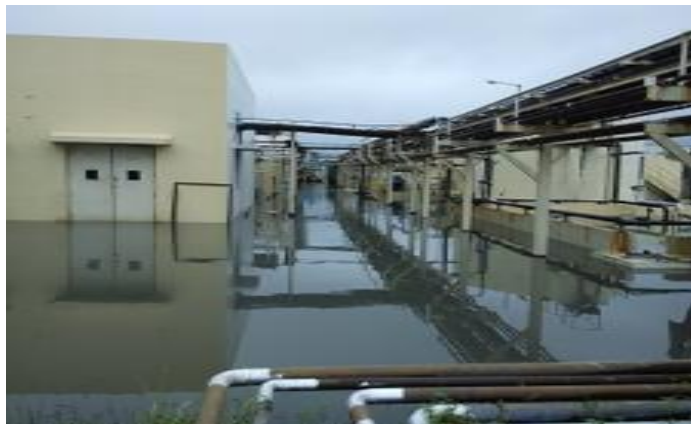
Water intrudes into factory
