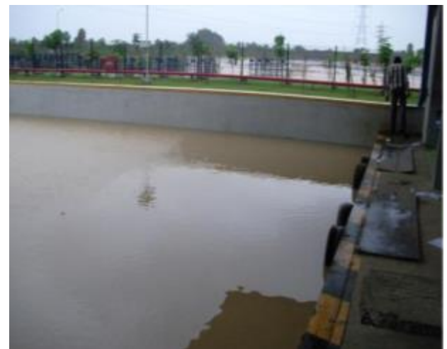
Water logging at dispatch yard
